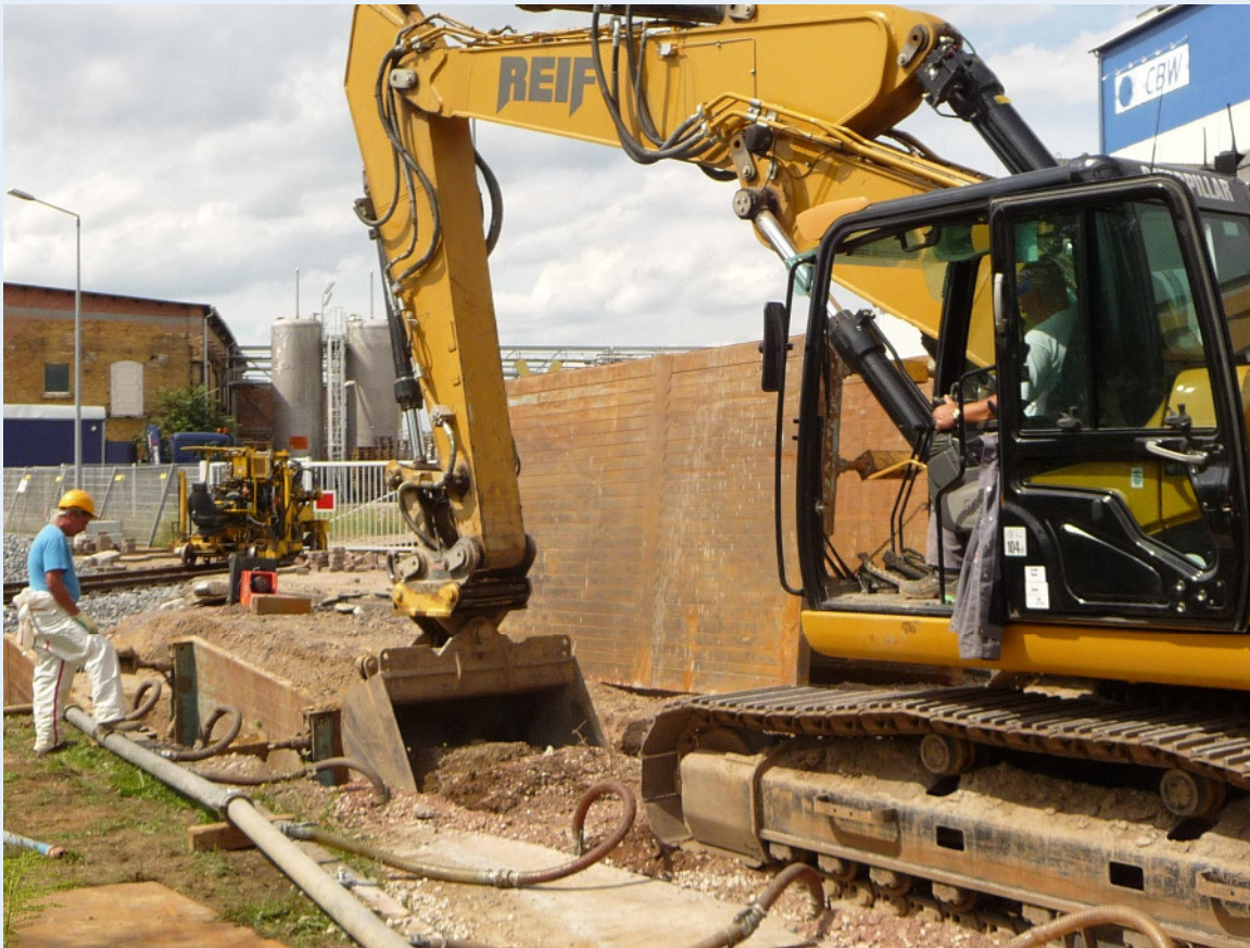
Replacing old sewer pipes in Hauptstrasse area
